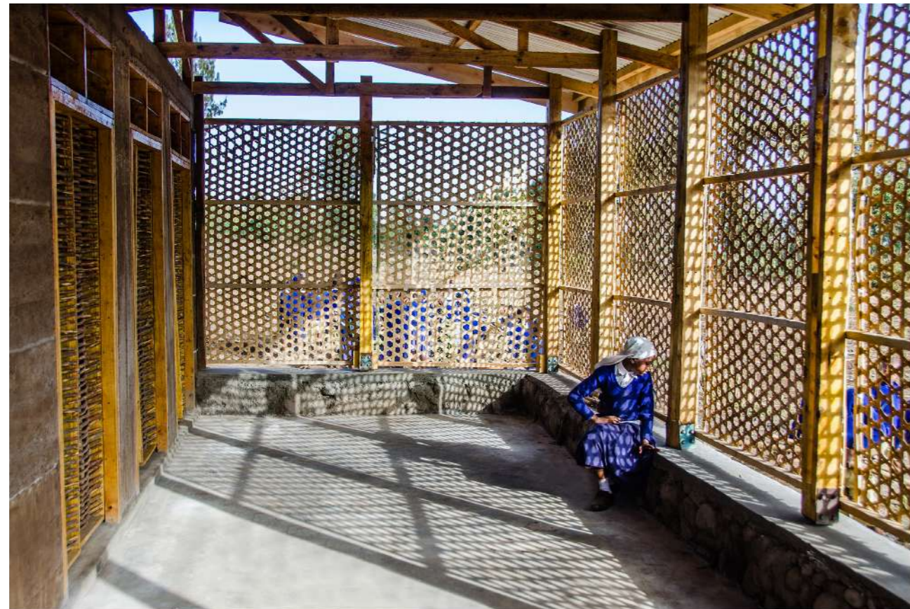
View of the verandah with the sun penetrating through the webbed bamboo
