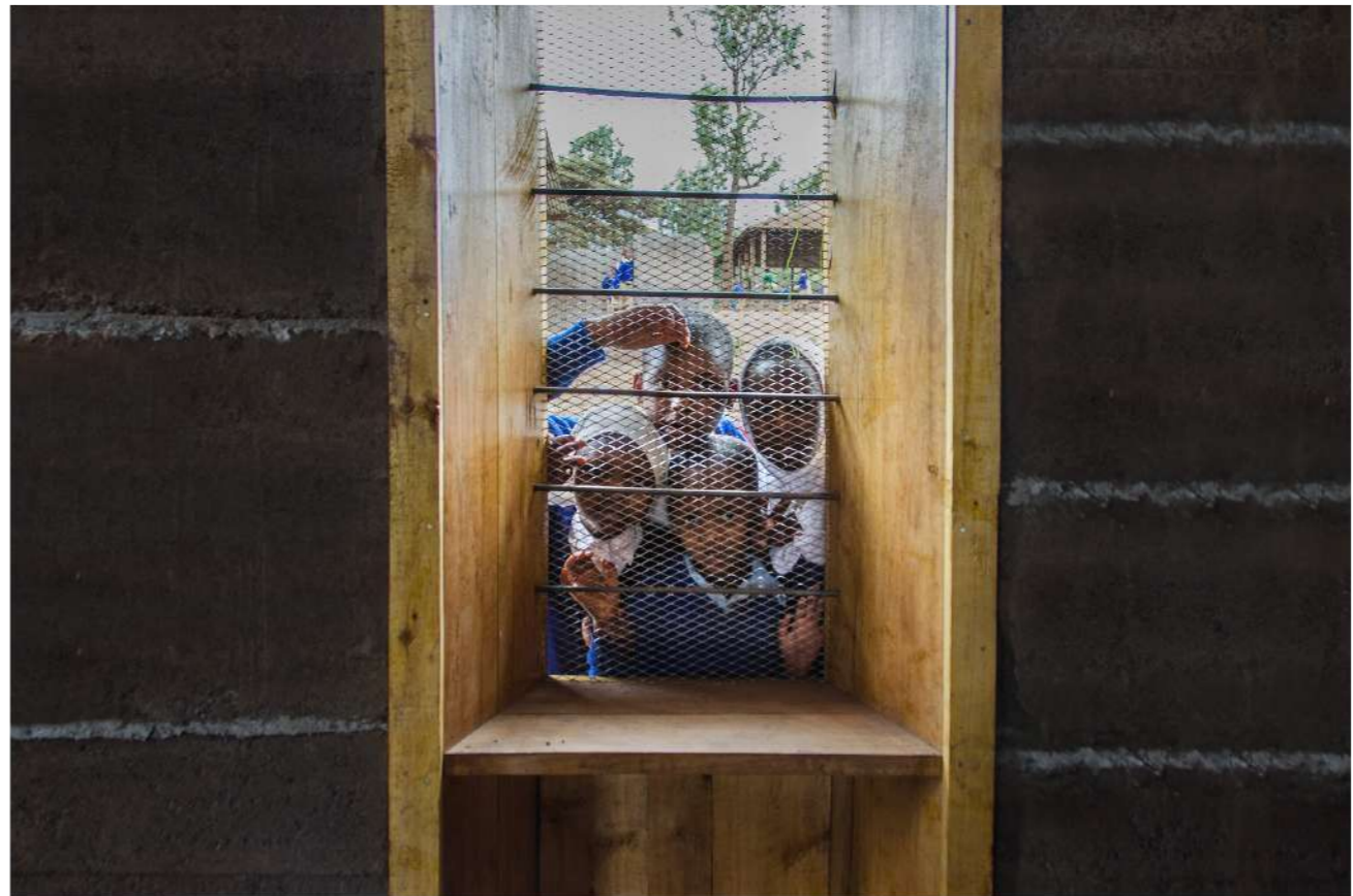
Detail of a window embedded in the earth wall
